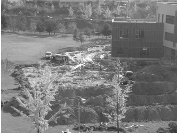
Figure 5. Trenches and double U-tubes for borehole heat exchanger for Earthquake Research Center building at KIGAM.
